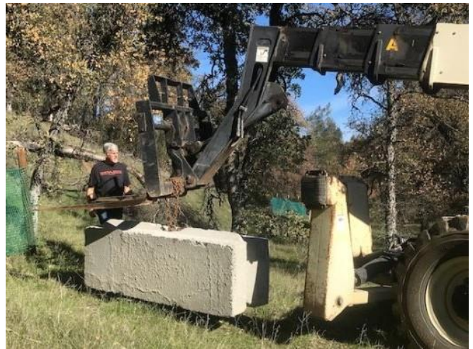
Jim Milestone directing placement of barrier. Photo by Bill Kuntz.
